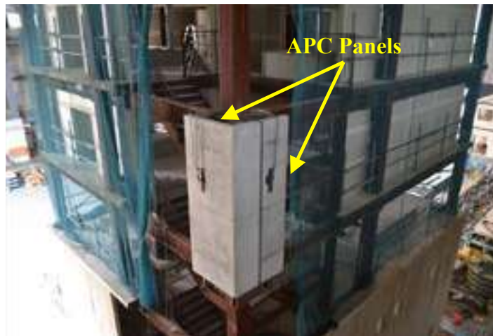
Figure 2.4. Upper stories of the E-Defense test building and APC panels
