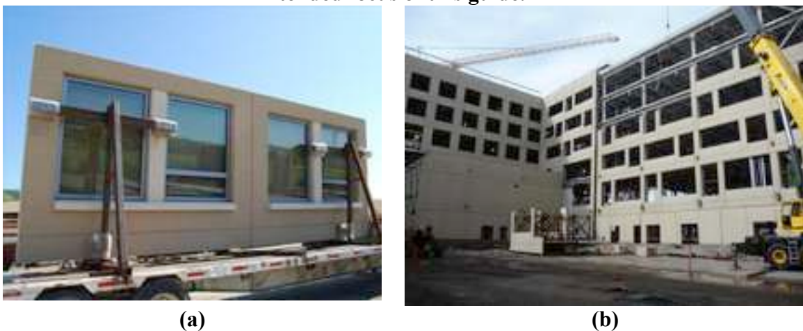
Figure 1.2. Examples of typical precast concrete cladding systems installed in the field: (a) punched panel system in transport and (b) u-shaped panels during installation.
