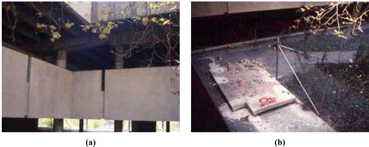
Figure 2.2. APC panel (a: as installed before) and (b: fallen from a parking garage) at CSULA during the 1987 Whittier Earthquake. One person was fatally wounding (Arnold, 2009 after Taly, 1988).
