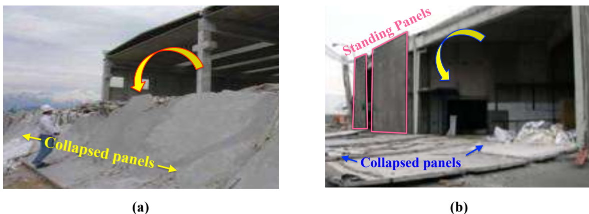
Figure 2.3. Photographs showing examples of collapsed panels after (a) the 2009 L'Aquila earthquake (Miyamoto International, 2009) and (b) the 2010 Chile earthquake (Gosh and Cleland, 2010)
